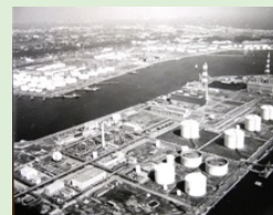
Minami-Yokohama Thermal Power Station
