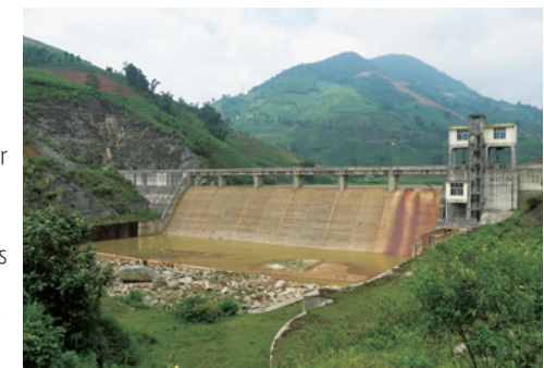
Coc San hydroelectric power station dam
