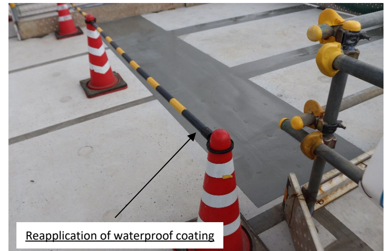
Waterproof caulking damaged by fieldwork (rubbing hoses) and footsteps
