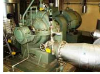
Turbine auxiliary cooling system
