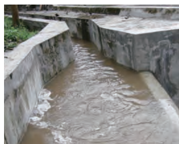
Power generation facility (sand basin)
