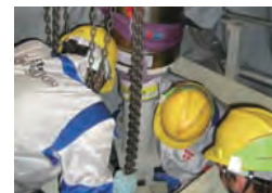
Seismic reinforcement of pipe supports (Unit 3)
