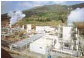
Hachijojima geothermal power plant (3,300kW)
