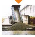
Concrete is used for roadbed material, iron reinforcement recycled as material for steel.
