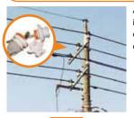
Attached to utility poles, insulators are made of ceramics that do not conduct electricity.
