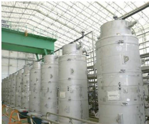
High-performance multi-nuclide removal equipment (absorption towers)
