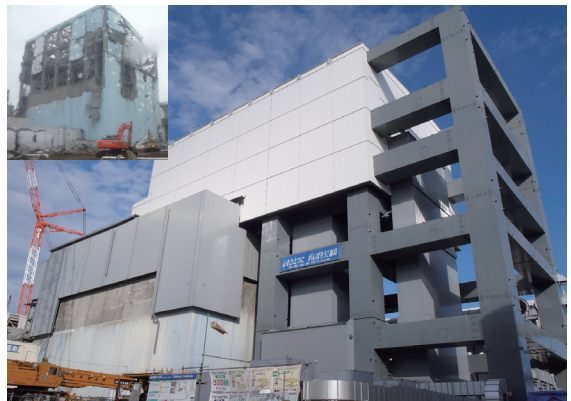
The extended structure and covering installed onto Unit 4 reactor building for the removal of fuel (Left above: Unit 4 reactor building immediately after the nuclear accident in March 2011)
