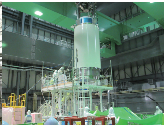
Removing fuel from the spent fuel pool of Unit 4
