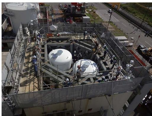
Installing iodine filters as part of above-ground filtered vent equipment of the Kashiwazaki-Kariwa Nuclear Power Station Unit 7
