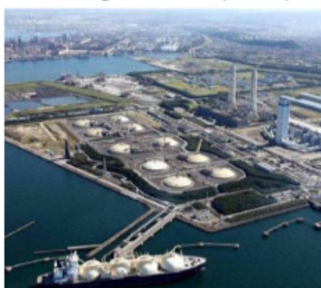
(Futtsu Thermal Power Station)
