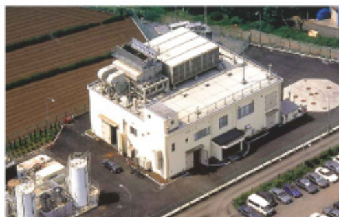
privately-owned electrical power facility
