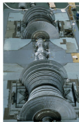
Steam turbine Taking off the cover for maintenance
