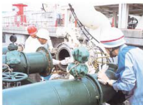
Careful connection of petroleum receiving equipment
