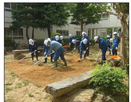
Simplified decontamination work in a school courtyard
