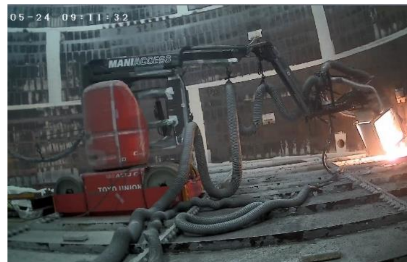
Using lasers to decontaminate a tank in E area (May 24, 2022)
