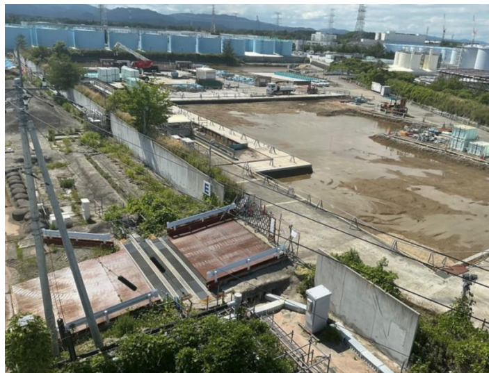
After dismantling D1 tank in E area (June 15, 2026)
