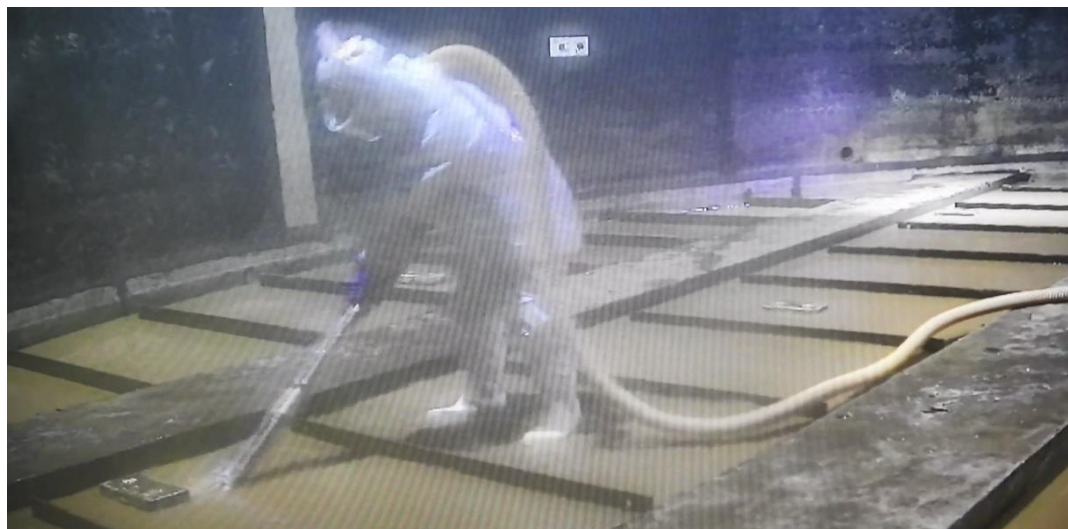
Cleaning the inside of tank D1 in E area (December 24, 2025)
