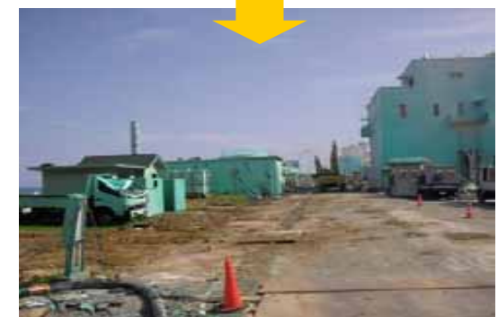
Removal of rubble
