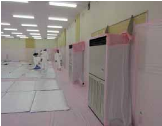
Inside the rest place in former Emergency Response Room
