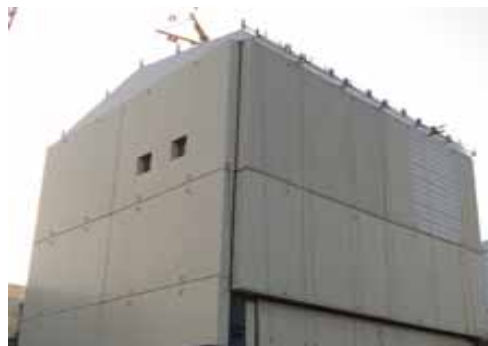
Unit 1 reactor building cover installation
