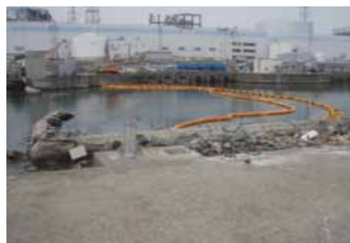
Silt fence installation
