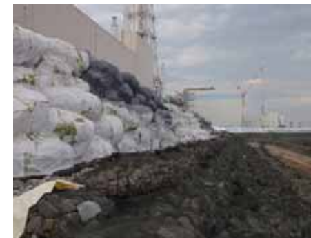
Installation of temporary tide barrier
