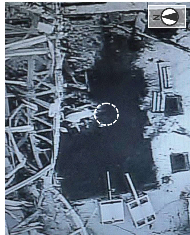
After steel truss debris removal (Photo taken on February 6, 2013)
