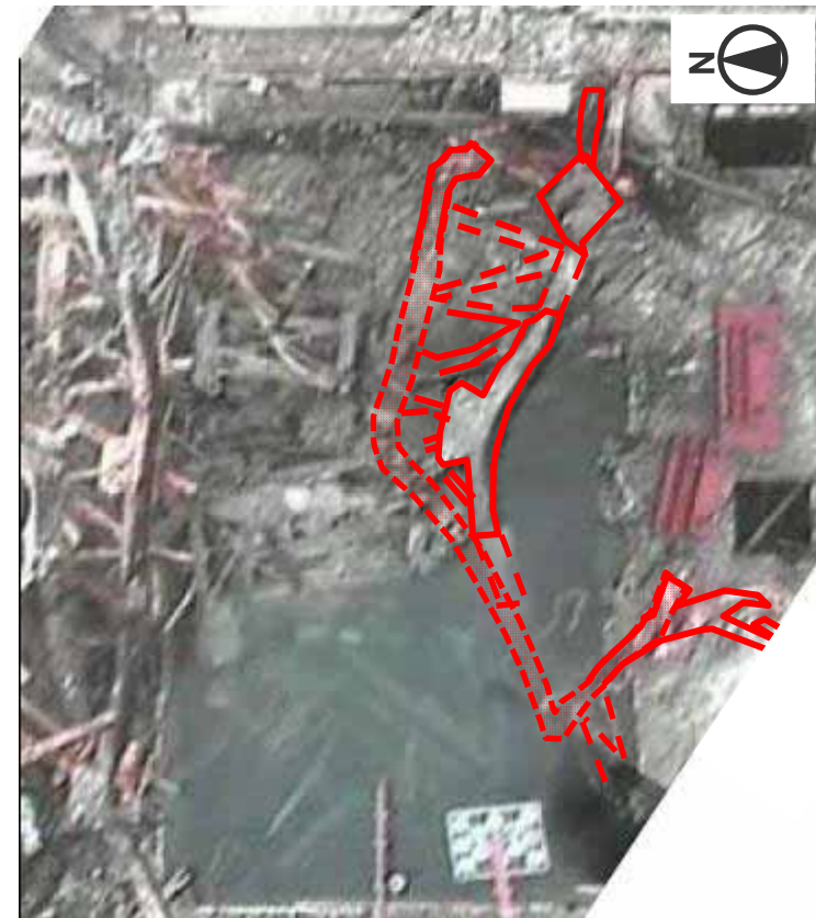
Interfering debris (After removal)
