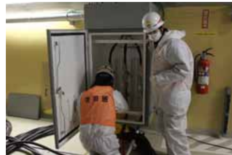
Making connection with the cable connection box (Unit 2)
