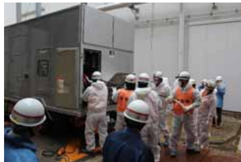
Pulling out cable from a power supply car (Unit 2)
