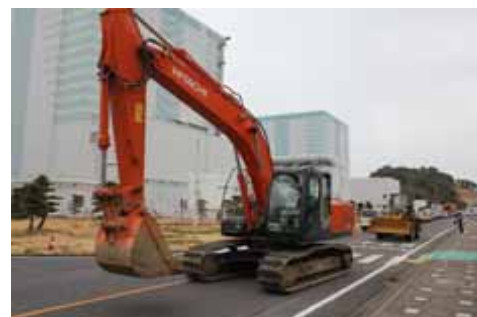
Checking the access route at the site (around the Reactor Building)
