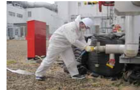
Transferring water to the Reactor Building (Unit 2)
