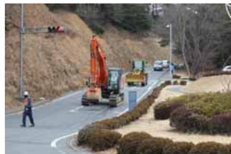
Heavy machinery heading to the site
