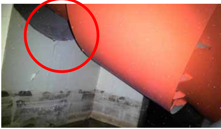
Edge of the vent pipe sleeve
