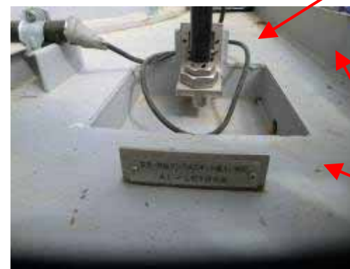
(Example) Leakage detector installed in the equipment skid
