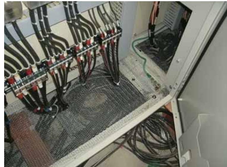
Implementation of countermeasure against small animals (installation of entry prevention net)
