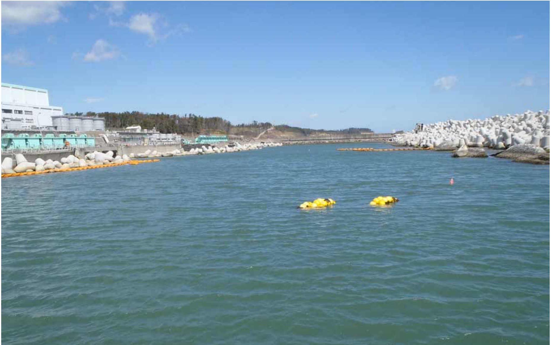
Condition of the silt fence on Units 5/6 side
