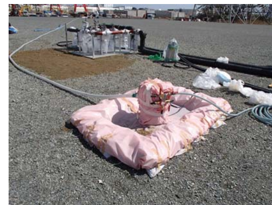
Installation of the pump at underground reservoir No. 3 (photo taken on April 13)
