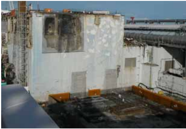
(1) Before the steel frame construction was started (December 18, 2012)
