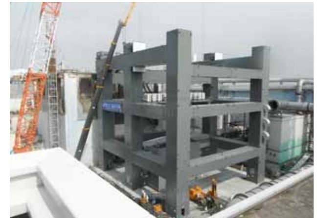
(3) Completion of the third layer of the steel framing (March 13, 2013)
