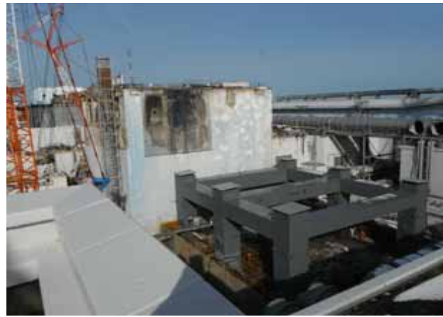
(2) Completion of the first layer of the steel framing (January 14, 2013)
