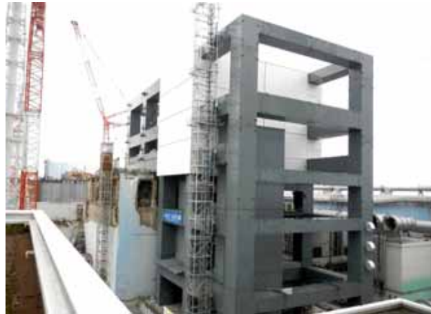
(5) Completion of the steel frame construction (May 29, 2013)
