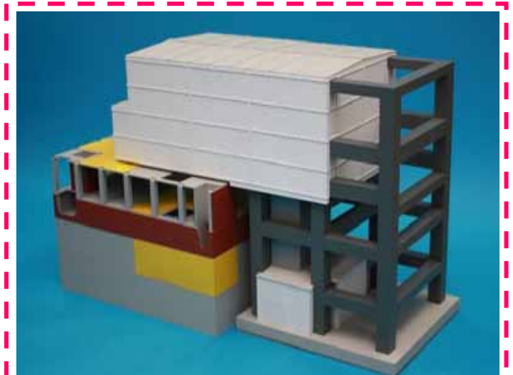
Simulated image of the cover to be installed for fuel removal
