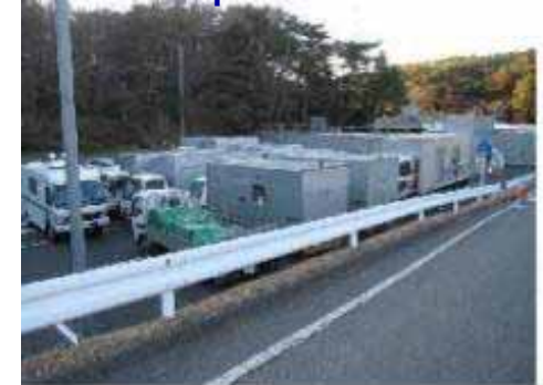
Replacement of electric motors
