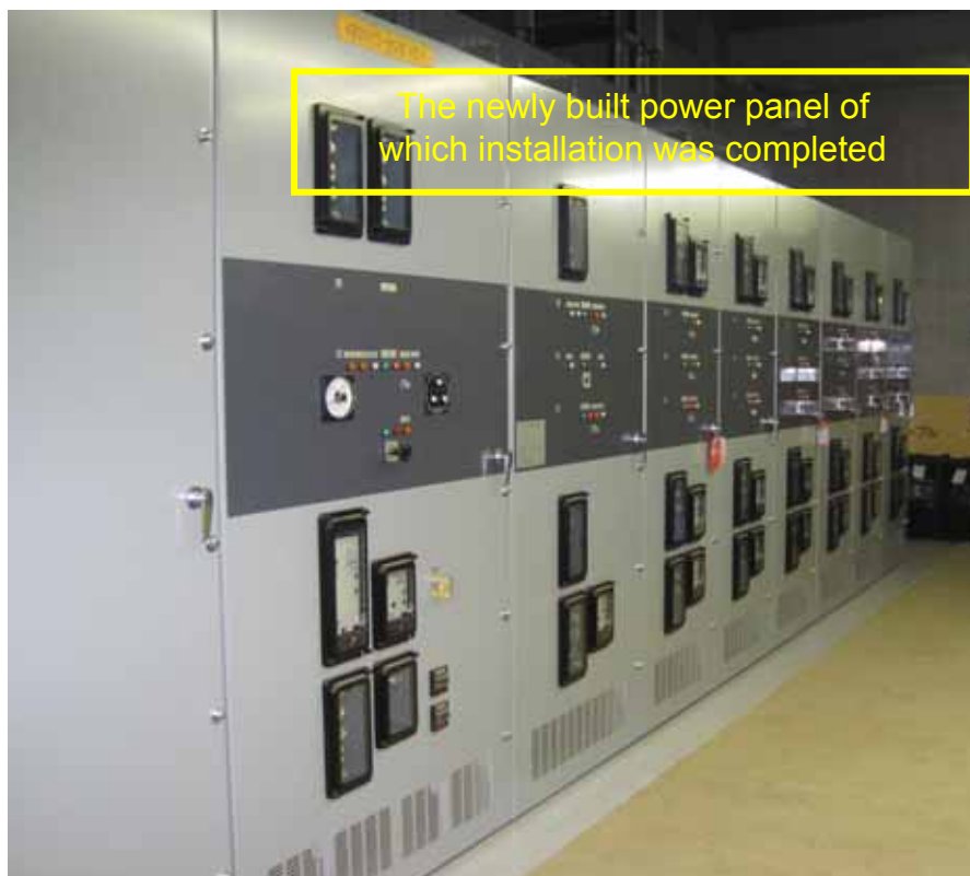
(After restoration work)
