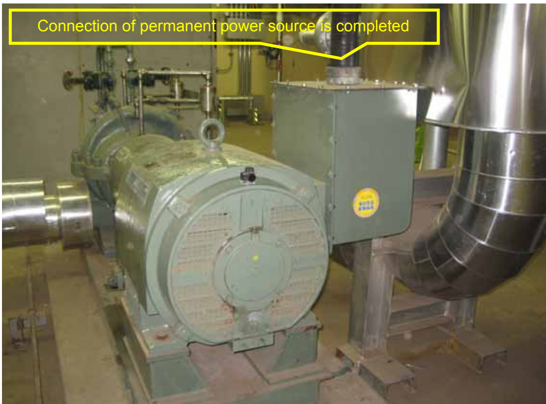
(After restoration work)
