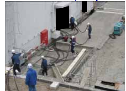
Installation of temporary cables
