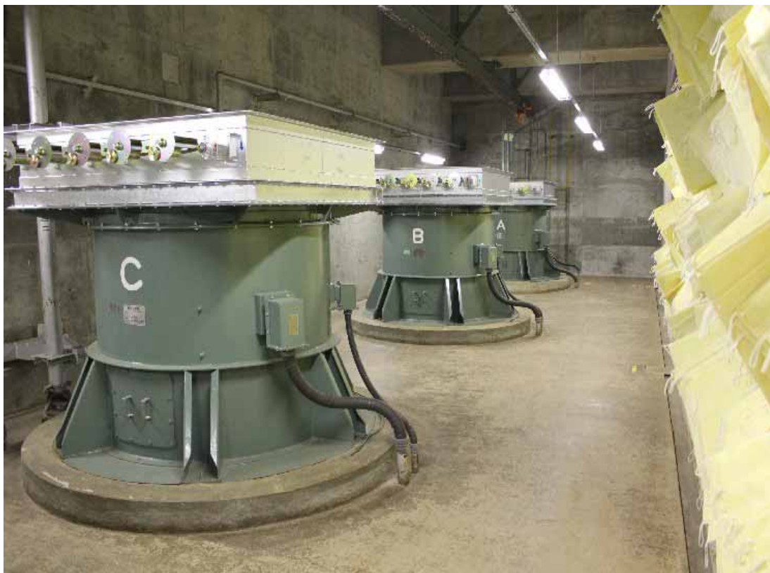
(After restoration work)
