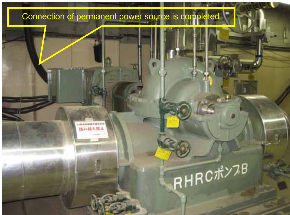
(After restoration work)
