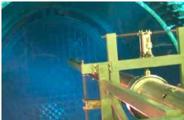
Extracting and lifting of fuels inside the reactors
