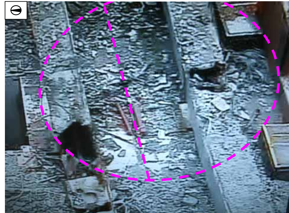
Condition around the shield plug (Photo taken by TEPCO on July 23, 2013)
