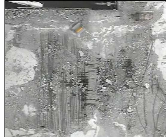
Photo ②: Reinforcing bars exposed due to damage to the upper end of concrete
