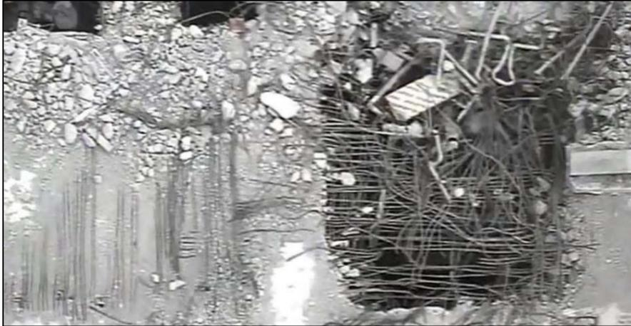
Photo ①: Damage to the floor slab
