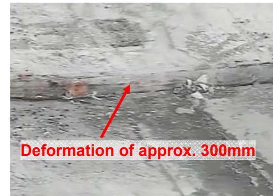
Photo ①: Deformation state of the shield plug
