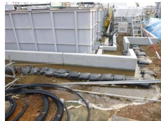
Leakage status (③ area)
