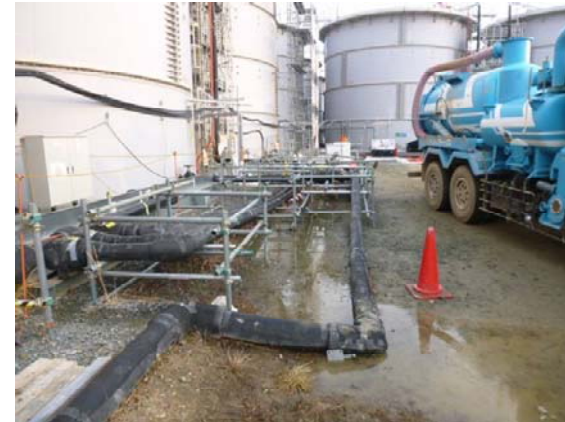
Leakage status (① area)
