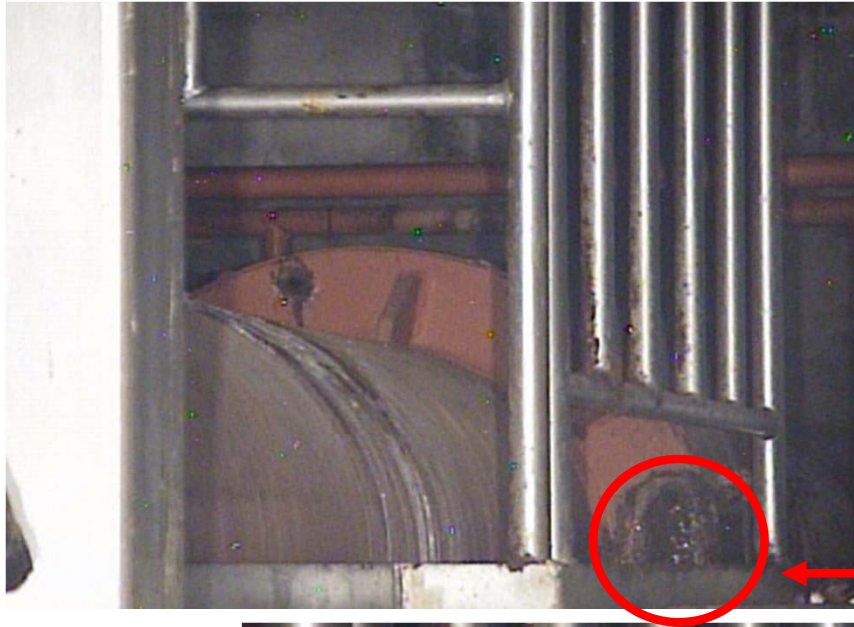
Flexible joint (opposite side of PCV)
