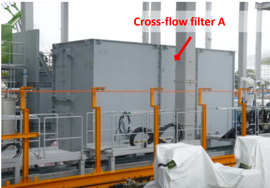
Cross-flow filter (photo taken on Aug 17 2014)
