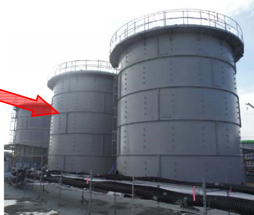
Rainwater receptacle tank No.2
