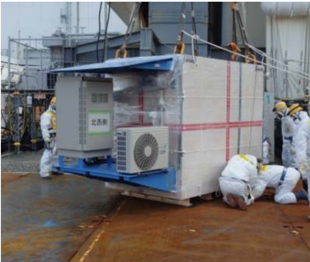
Image 3: Installation of Detector-1 (North West side)
