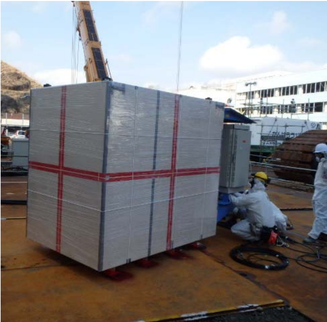
Image 5: Cable connection to Detector-1 (NW side)
