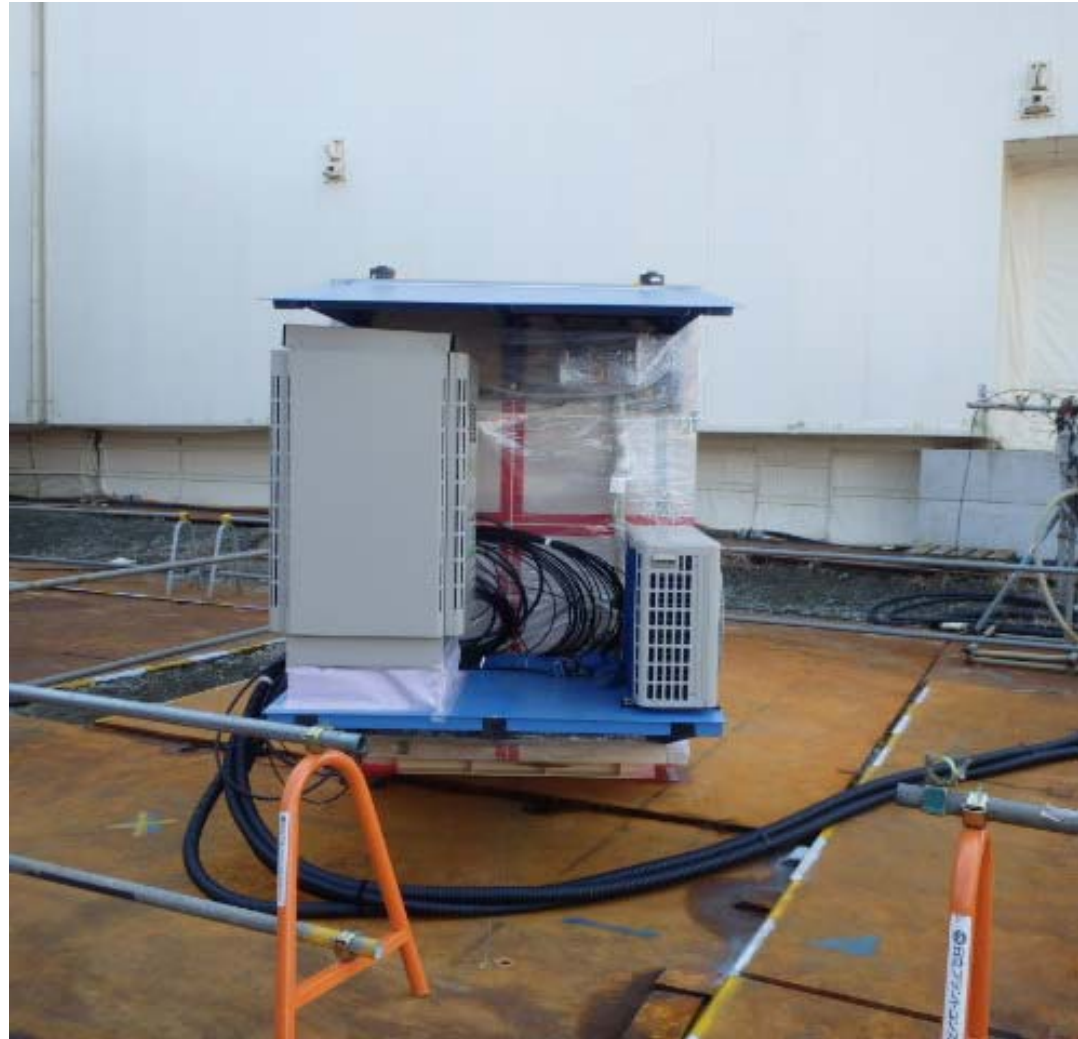
Image 6: Detector-2 (North side) installation completed
