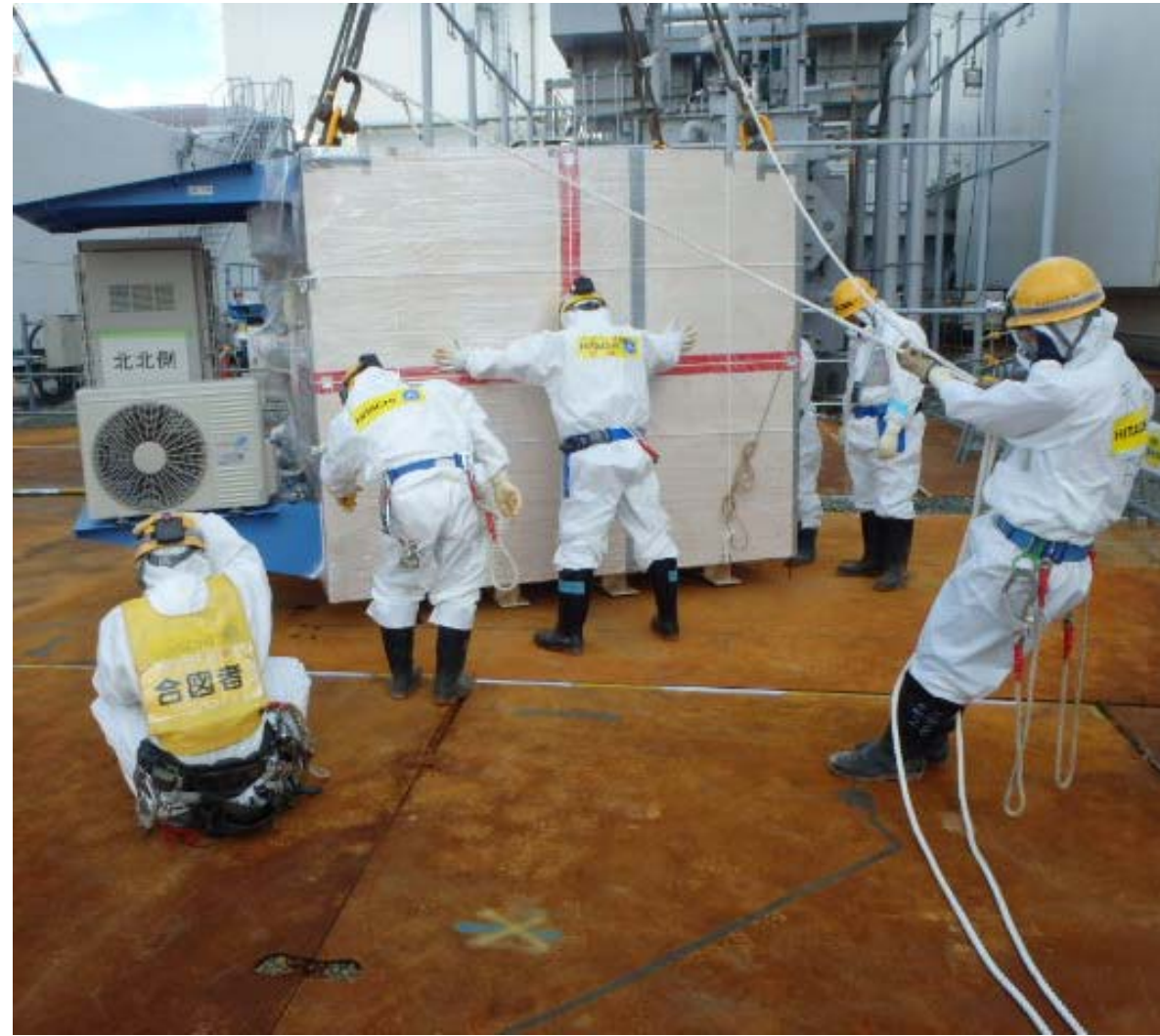
Image 2: Installation of Detector-2 (North side)
