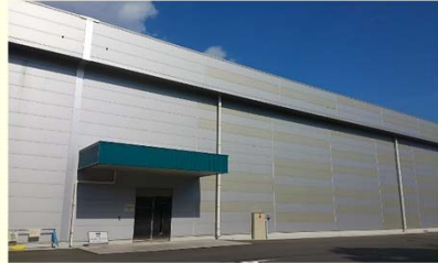
<External appearance of new Administration Office Building>
