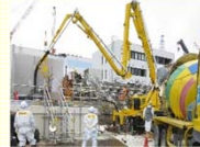
<Removal of contaminated water>
