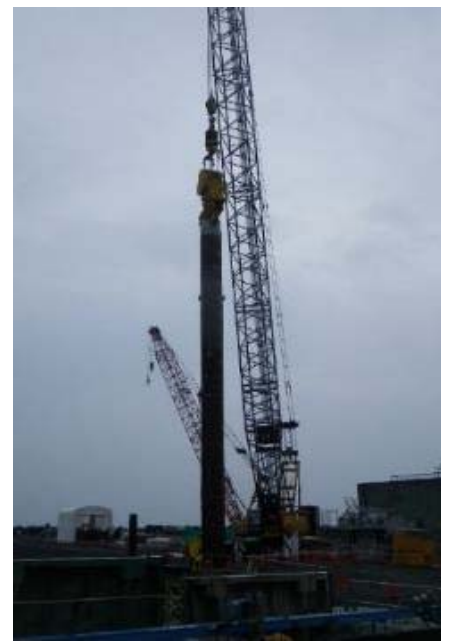
Placing steel pipe sheet-piles (1 st step)
