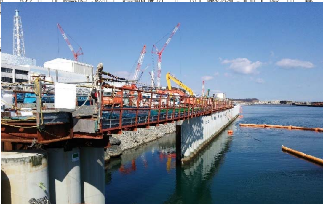
Seaside impermeable wall closing point: The open space for 9 steel pipe sheet-piles to be placed (approx. 10m extension)
