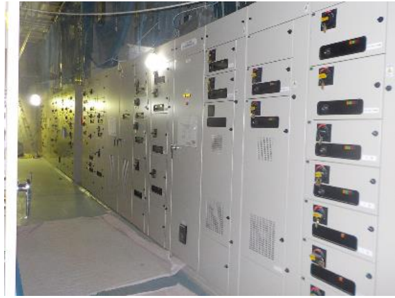
Electric panel room
