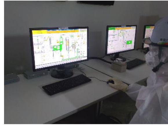
Control room under trial operation
