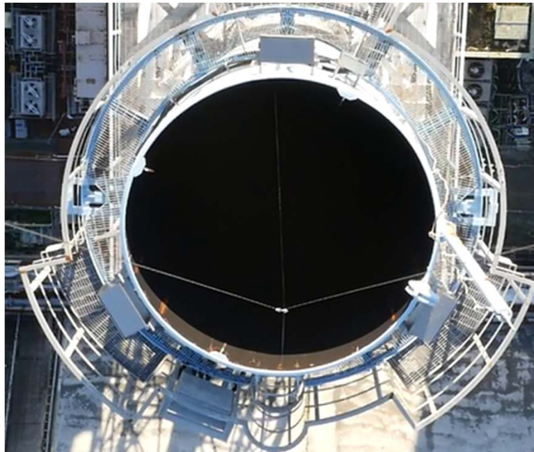
Exterior of the exhaust stack
