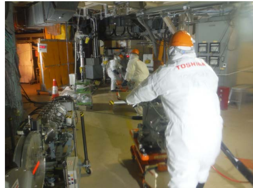
Inside the Unit 2 Reactor Building
