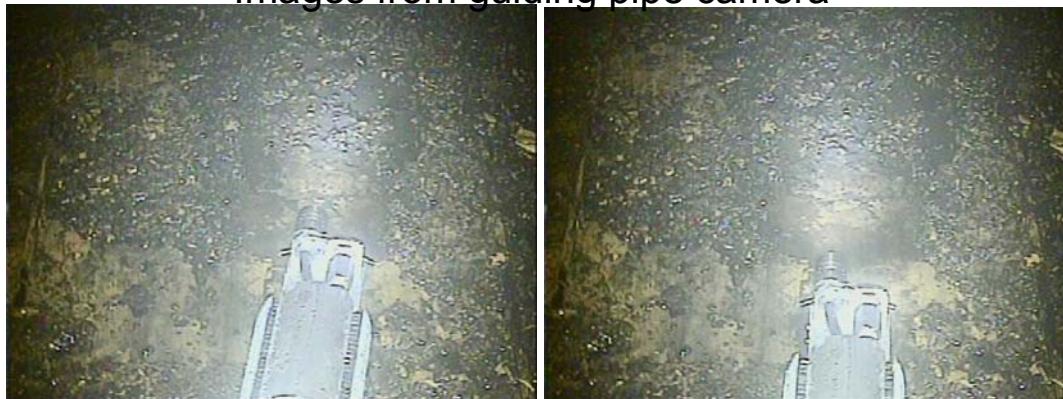
Before the removal
