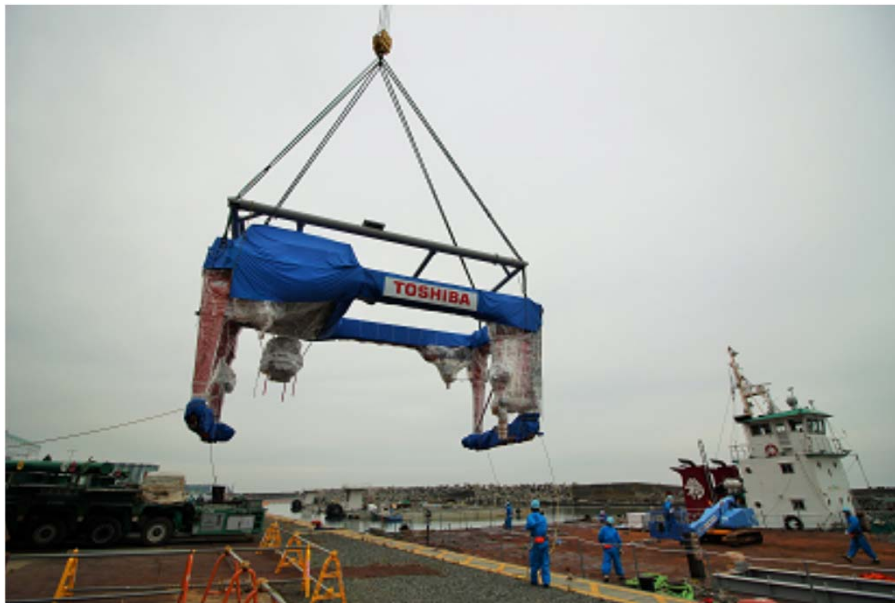
Fuel handling machine (being carried in the site from the sea)
