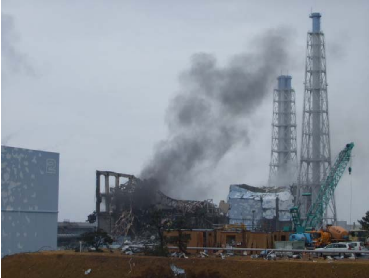
Apparent condition of Unit 3 after explosion (page 35)
