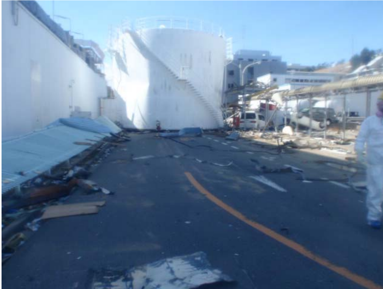
Flowed tanks by tsunami (page 11)
