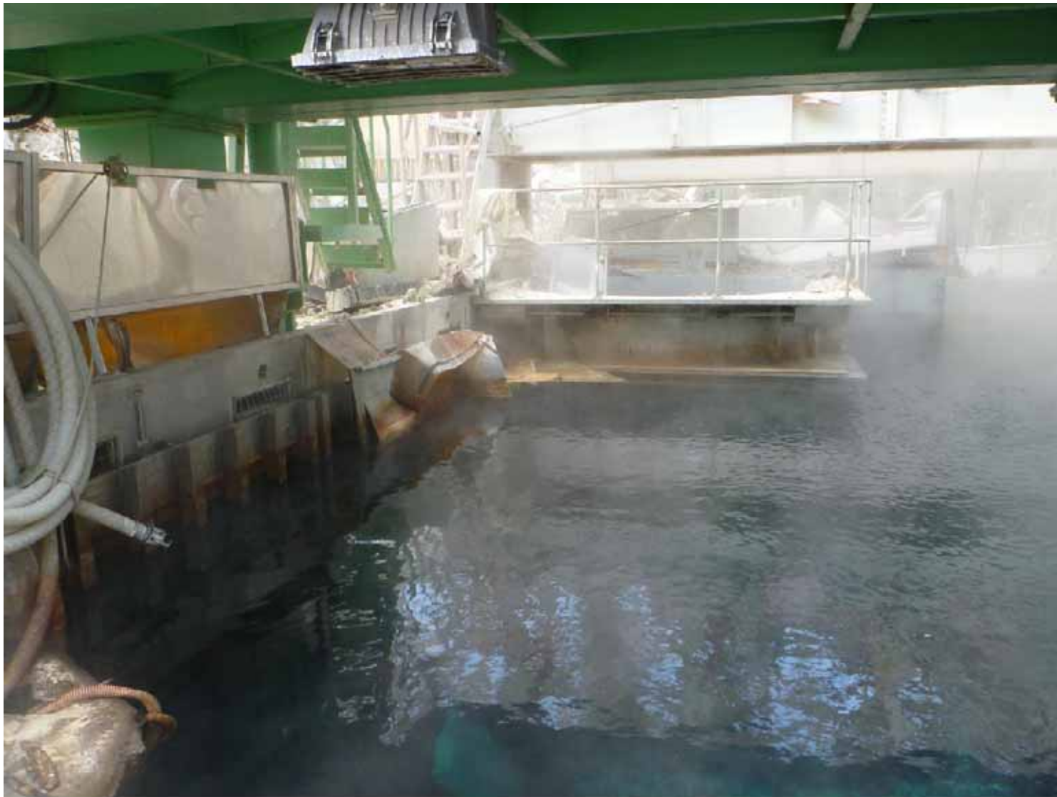
Spent Fuel Pool in Reactor Building (5th floor), Unit 4, Fukushima Daiichi Nuclear Power Station
