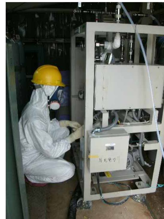
1F Unit 2 PCV temporary gas sampling instrument
