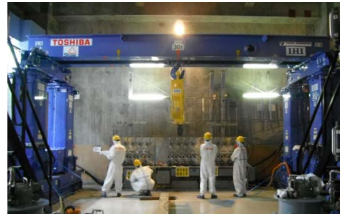
Crane for vessel replacement August 2, 2011 Photo by partner company
