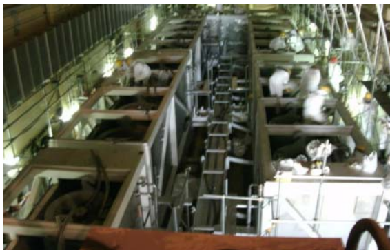
Kurion Cesium adsorption apparatus June 8, 2011 Photo by TEPCO
