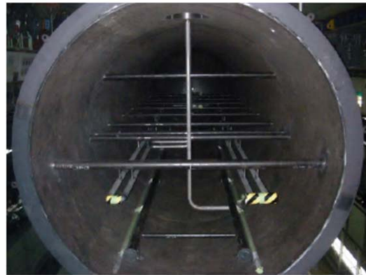
Iron storage tank for sludge in progress (Inside)
