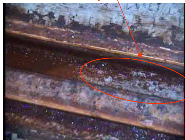
Gutter of rails, after wiping
