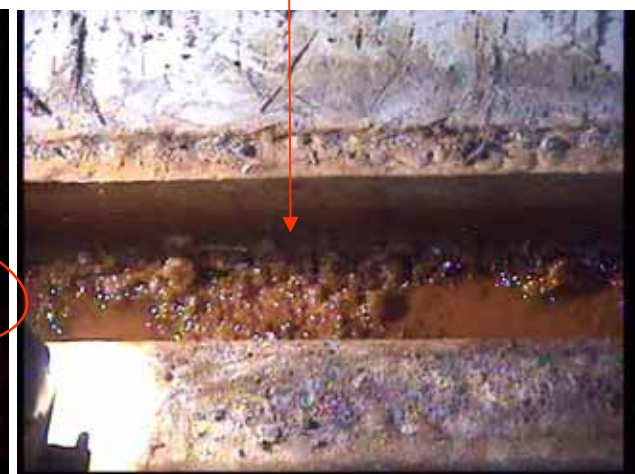
Gutter of rails, after wiping
