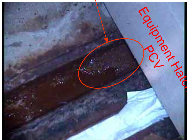
Gutter of rails, proximity of Equipment Hatch, PCV
