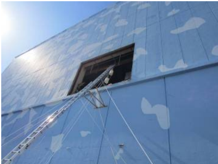
Measurement at the blowout panel
