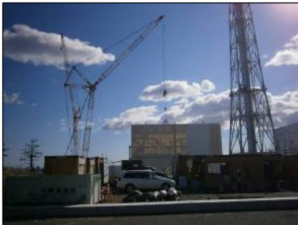
Measurement at the upper side of the reactor building
