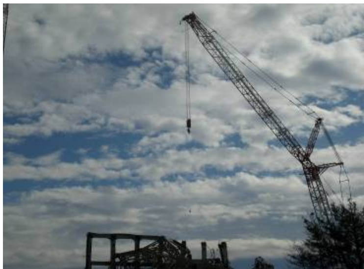
Measurement at the upper part of the reactor building
