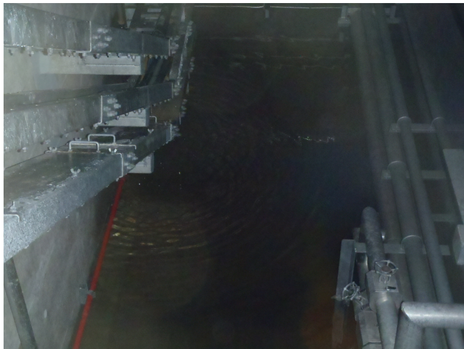
【photo 】 Accumulated water in the trench
