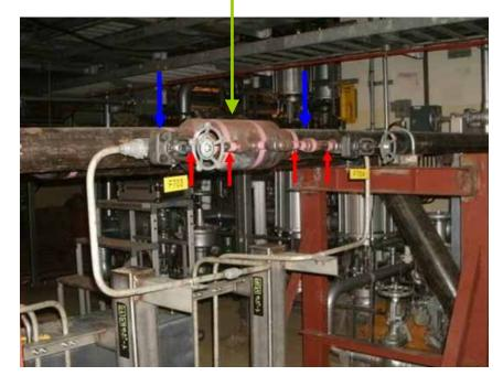
: Primary side pipe cuttings : Instrumentation pipe cuttings
