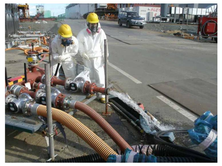
Start-up testing of the SFP water transfer pump (near the Main Office Building) Photo taken on January 26, 2012 and presented by Tokyo Electric Power Company, Inc.
