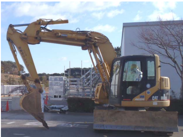
Scraping the road
