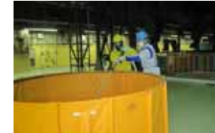
Transporting the water to the reactor building (temporary tank) (Unit 1)
