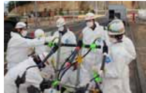
Connection of power cables (Unit 3)
