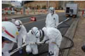
Connection of power cables (Unit 3)
