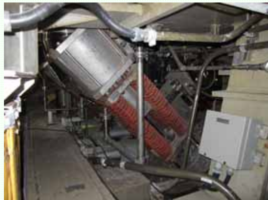
Main Steam Isolation Valve ( February 22, 2012 )
