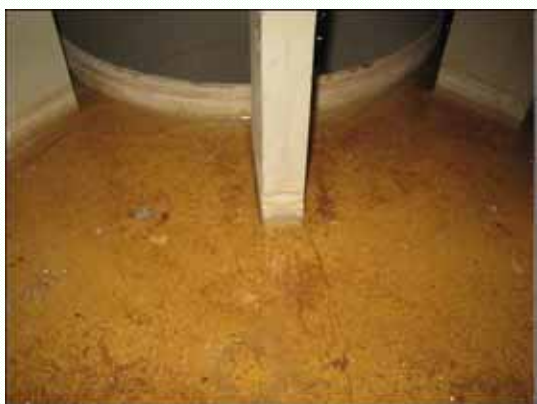
Puddle ( Diaphragm Floor ) ( December 27, 2011 )
