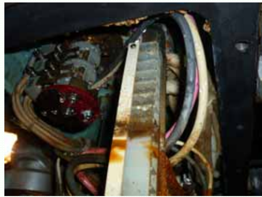
Retting of Terminal Box of Electrical Parts ( February 15, 2012 )
