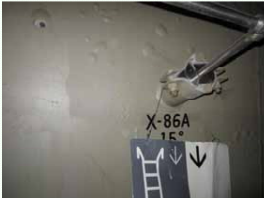
Peeling of painting on the surface of a wall (February 20, 2012)
