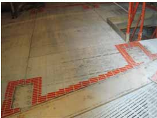
Exfoliation of Zinc Plating (Grating) (January 6, 2012)
