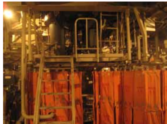
Primary Loop Recirculation Pump (A) ( February 2, 2012 )
