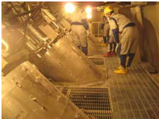
Main Steam Isolation Valve ( February 2, 2012 )
