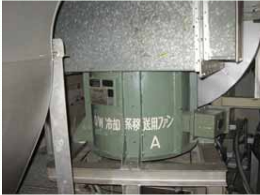
Drywell Cooling System Transfer Fan (February 8, 2012)
