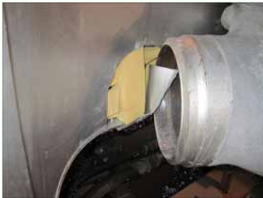
Separation of Lagging Material ( February 7, 2012 )
