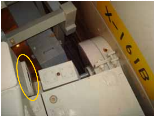
Crack on Weld Cap of Supporting Structure ( October 4, 2011 )
