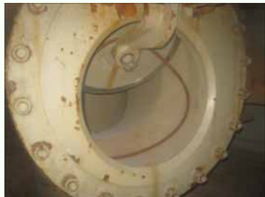
Rust on the Equipment Surface and Dislocation of Sheet Gasket (PCV Vacuum Breaker) (February 15, 2012)
