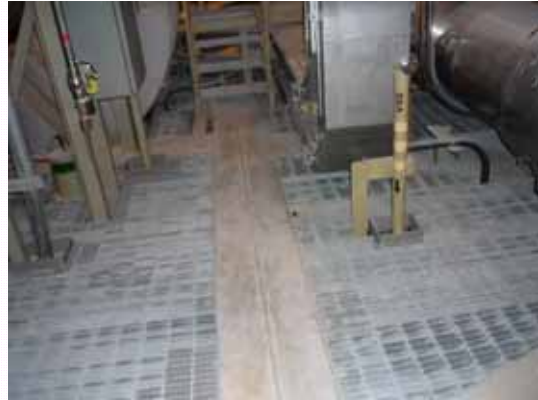
Exfoliation of Zinc Plating (Grating) ( September 6, 2011 )
