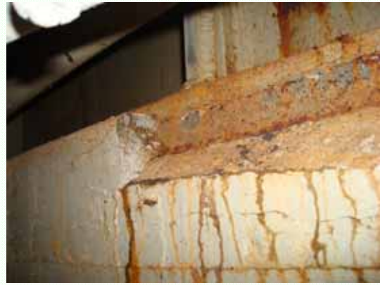
Exfoliation of Mortar (January 16, 2012)
