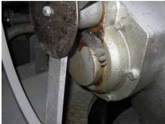
Grease leak from Valve Actuator ( February 20, 2012 )
