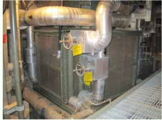
Drywell Cooling System Fan (February 8, 2012)
