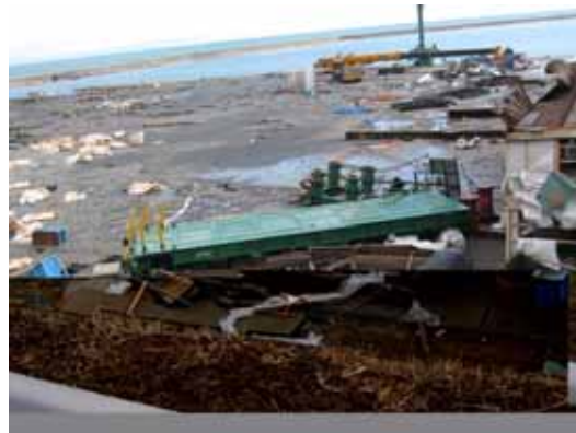
(2) Damage to the low area (Pickup area)
