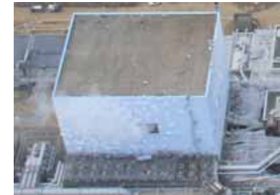
Opening the Unit 2 blowout panel
