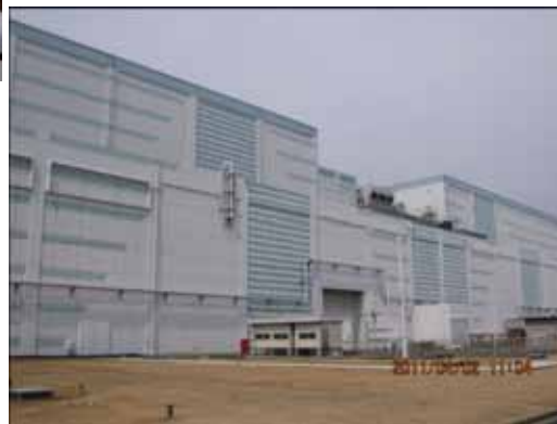
(3) No damage to Turbine Building of Units 3 and 4
