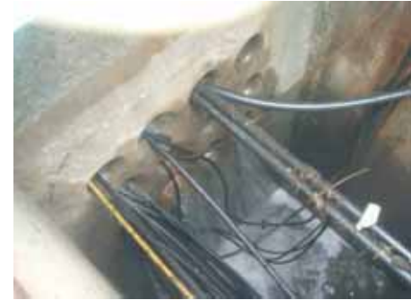
Situation in the pit near Unit 3 intake
