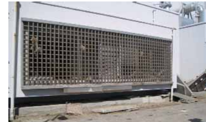
Outside of Unit 1 emergency air blower room
