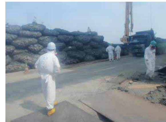
Installation work of temporary coastal barrier
