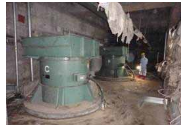
Inside of Unit 1 emergency air blow room
