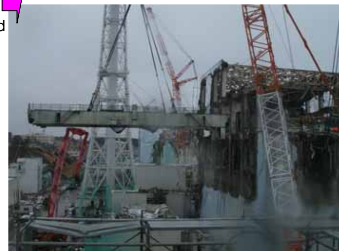
Removal of Unit 4 crane garter 2012.3.5
