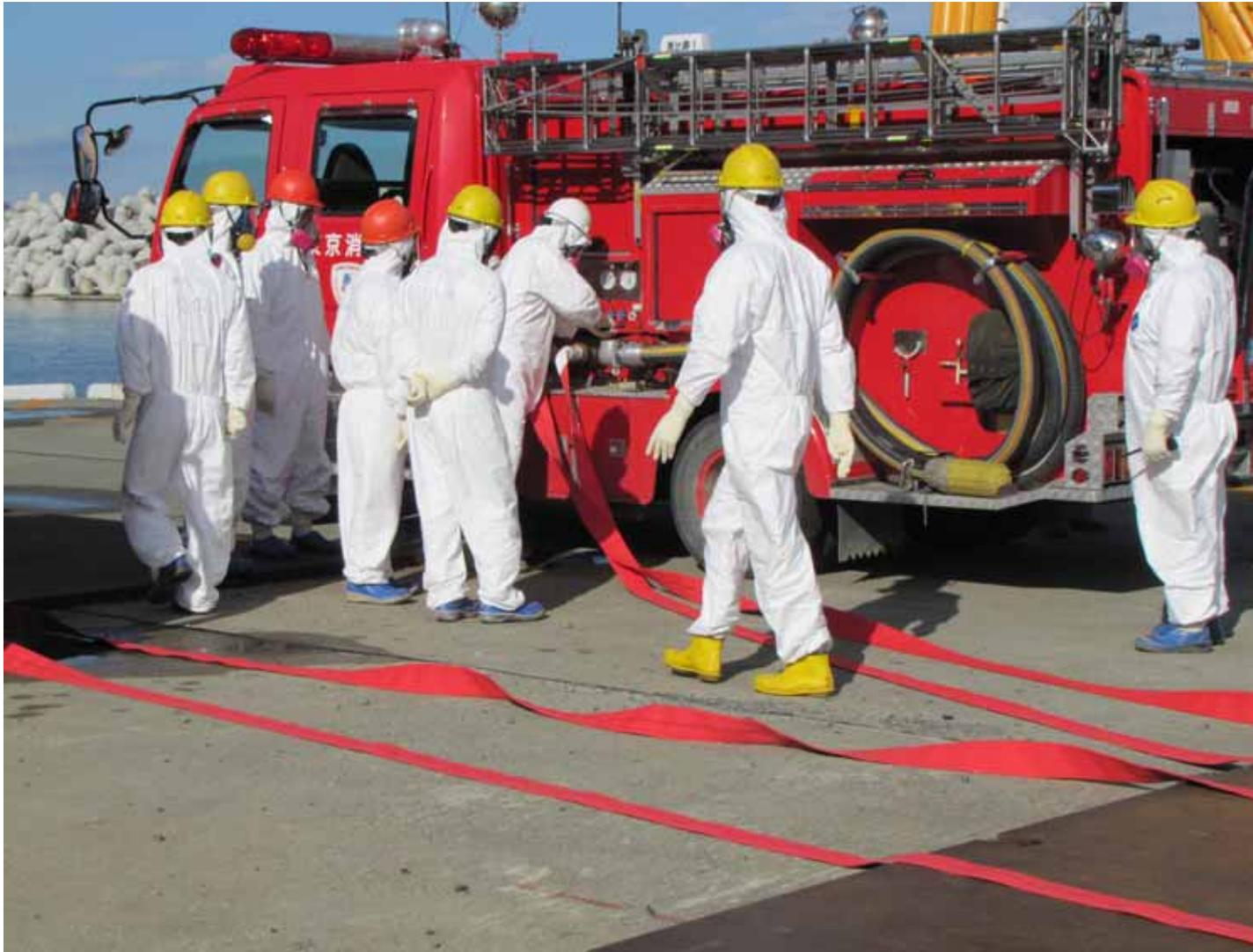
**Water injection to the reactor by using pump of fire truck
